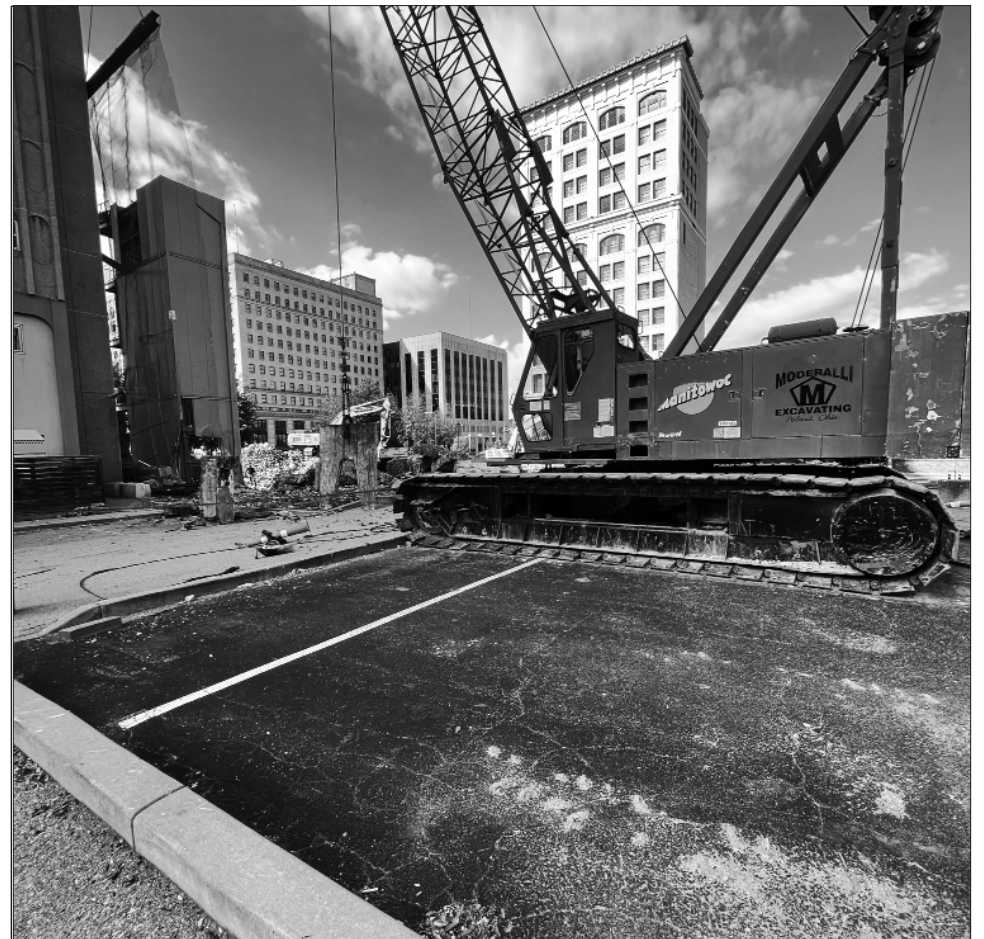
Demolition is set to be finished by the end of September.
